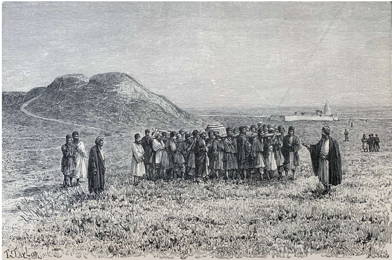
Transportation of a base of a column
